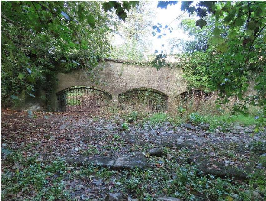
Photo 7 – southern elevation of old ford on Cootes Lane
