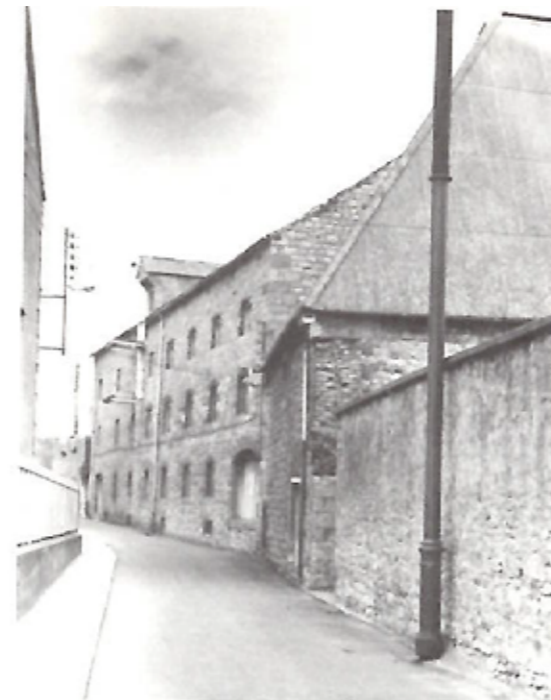
The Malthouse, Tilbury Place
