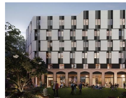
Apartments around open space
