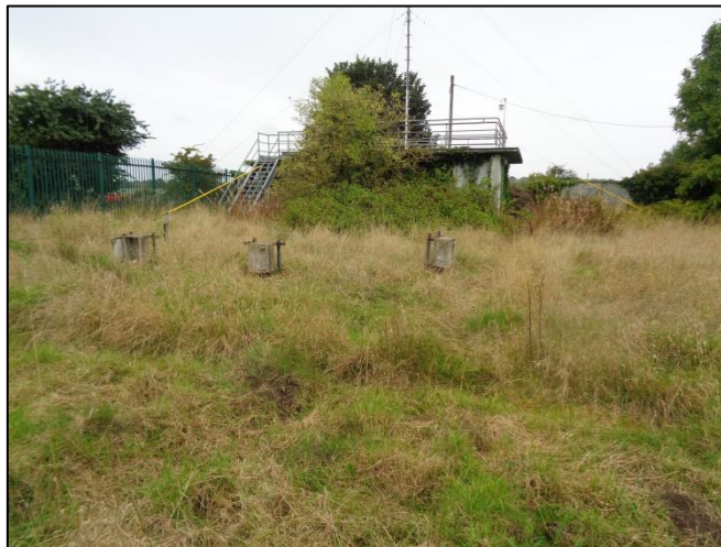
Pl. 9. Looking North at Site.
