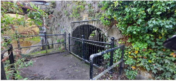
8. Northern opening to tunnel under Green's bridge
