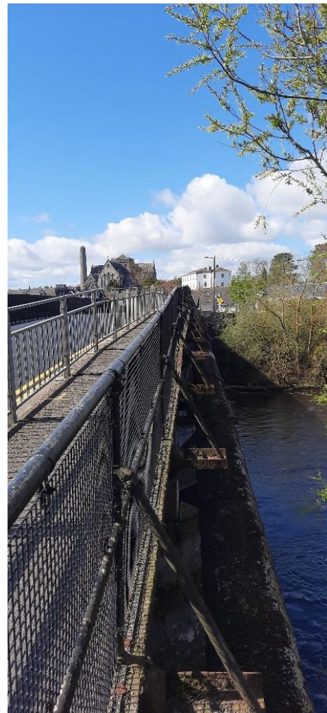
7. Extended walkway at side of Greens Bridge to North
