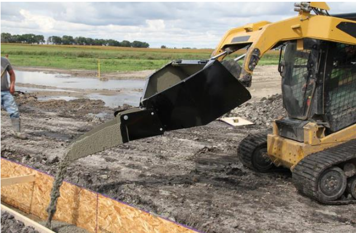
Figure 6 Concrete Funnel Bucket on Skid Steer Loader
