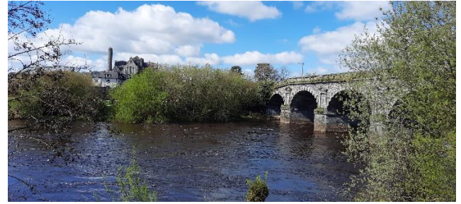
5. Greens bridge from south side
