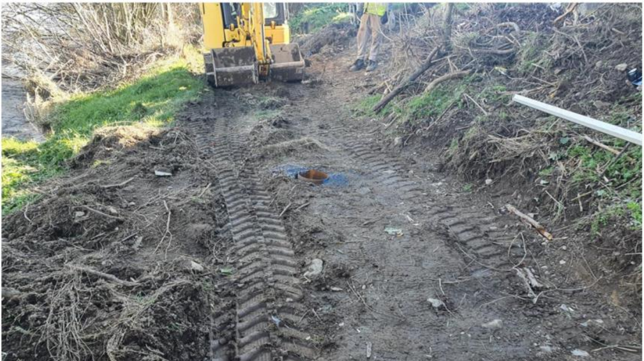
Figure 4: Photo of test pile
