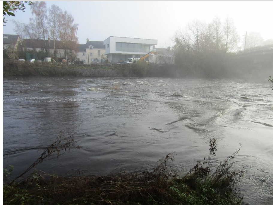
Plate 3 Showing water breaking in the River Nore where surviving piers of Greensbridge AH03 remains under the water, facing east.
