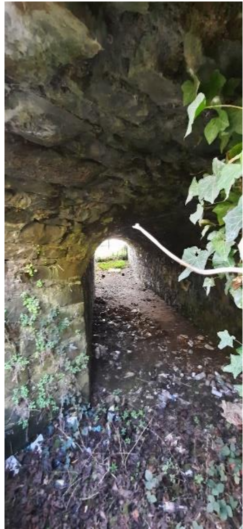
10. View through tunnel
