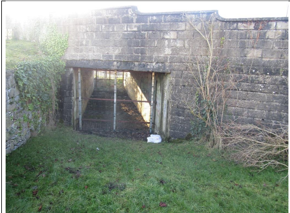
Plate 1 Showing existing stone arch of Greensbridge with tarmac path, facing south.
