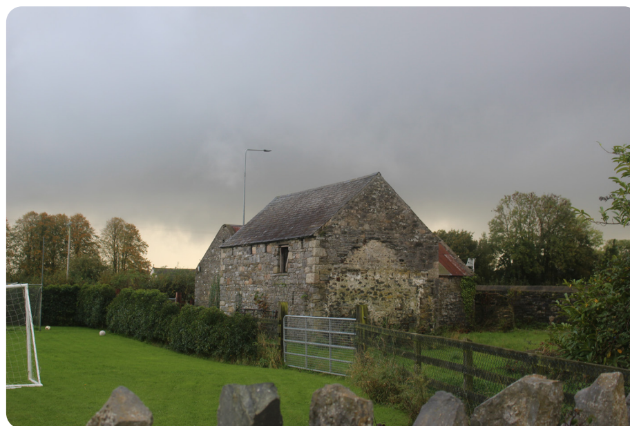
Figure 5.16: Derelict heritage farmhouse on intersection between St. Enda's terrace and R448.
