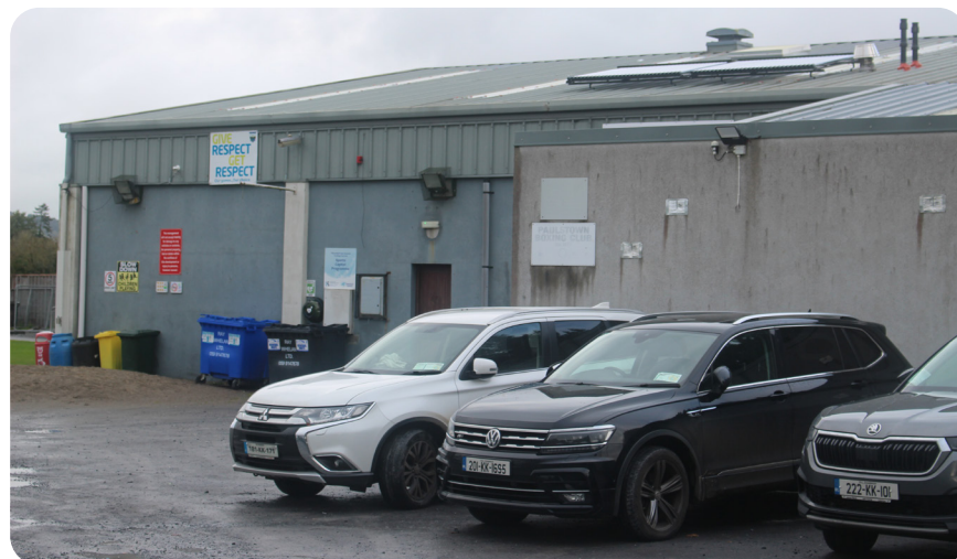
Figure 5.22: Paulstown Community Centre
