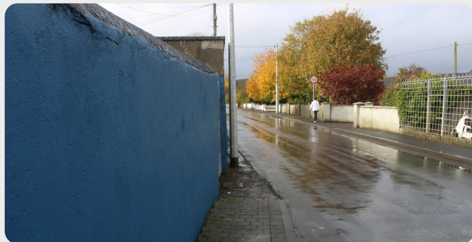
Figure 3.33: Pavement disappears along An Choill Rua
