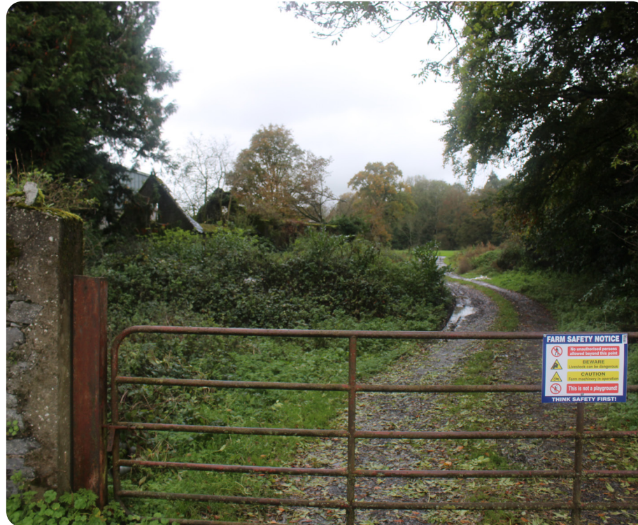
Figure 5.24: Derelict building in Paulstown
