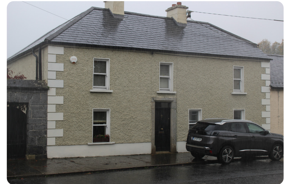
Figure 5.15: Building along Main St.
