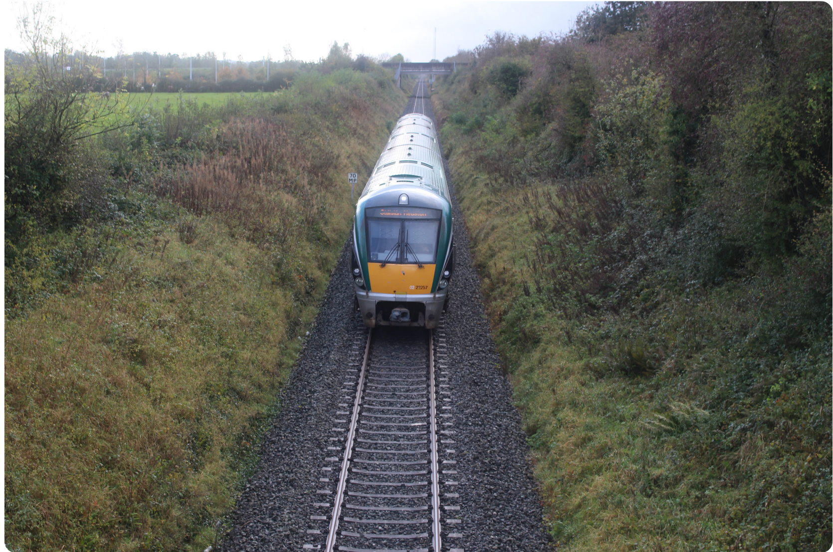
Figure 5.13: Railway along the western boundary of Paulstown.
