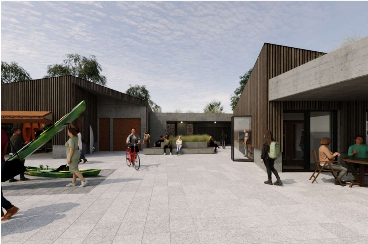
Figure 19: Proposed view from the site looking west highlighting the material palette – board marked concrete, accoya timber cladding, corten steel, green roofs and limestone paving
