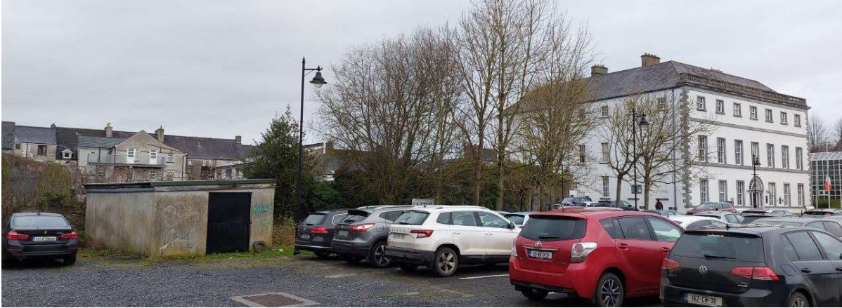
Figure 1 – Existing site within council carpark area. Maintenance store to left for demolition to accommodate new scheme
