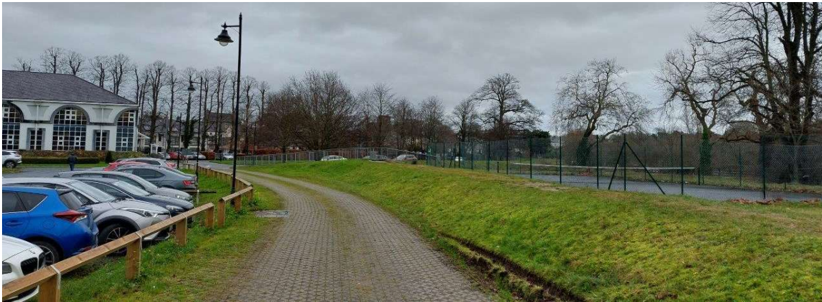
Figure 2 – Existing flood defence berm (right) & grasscrete access road alongside carpark. View looking towards Maudlin St.
