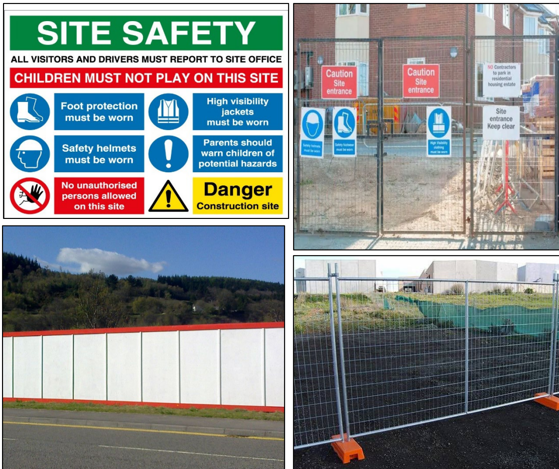
Figure 2.3: Examples of Signage and Fencing to Secure Construction Site
