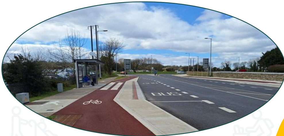
Similar bus bay, Newtown Road, Wexford Town
