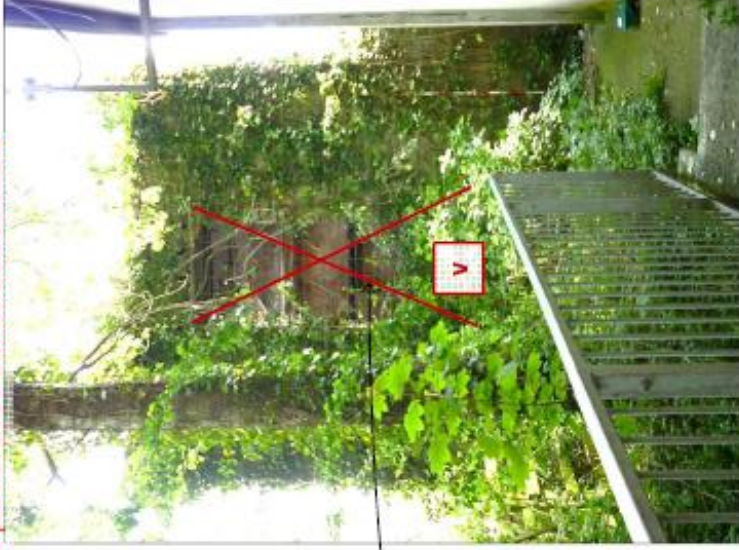
North elevation - vegetation to be close cropped
