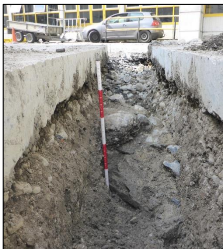
Plate 29 Monitoring ESB trench, culvert section 1
