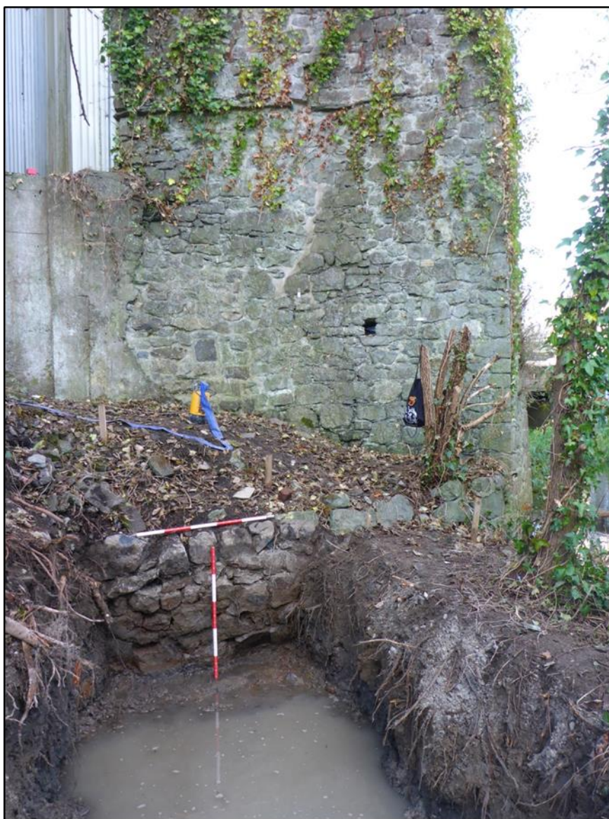
Plate 31 Revetment wall at Evan's Tower
