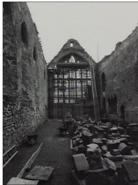
Plate 36 Work in progress to East Window
