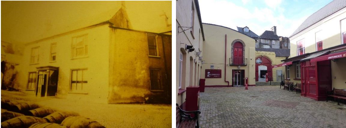
Plates 59-60 Visitor Centre showing Brew Masters House
