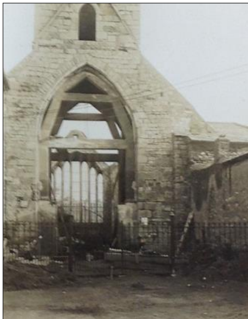
Plate 35 Northern elevation of Tower 1928
