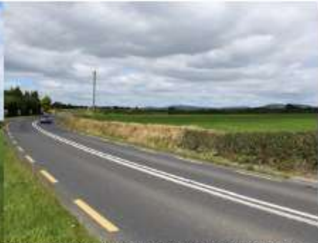
Pl. 10 Lands at Grange, looking northwest along the Magenta, Blue and Green route options.
