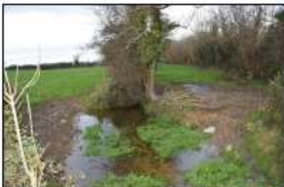
Plate 2 Skelptown 16 Stream (Segment Code: 16_10766) which crossed the existing N24 road, December 2017.
